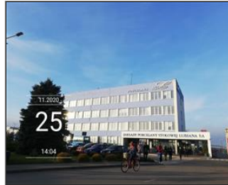
External photo(s) of the production unit(s) IMG_20201125_140415_1.jpg
