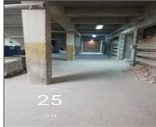
Photo of the inside of the main production hall IMG_20201125_134441.jpg
