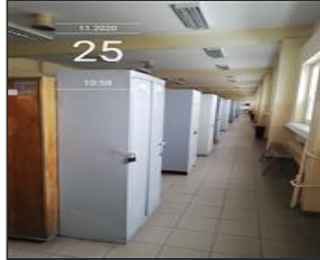
Photo of the sanitary facilities IMG_20201125_105813.jpg
