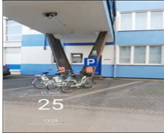
External photo(s) of the production unit(s) IMG_20201125_132936.jpg
